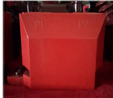
Resin current transformer
